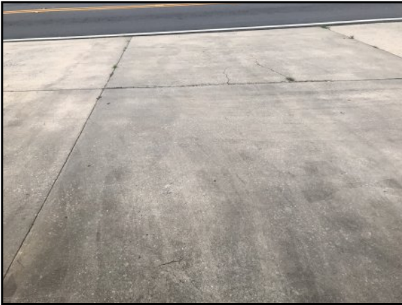
13 : De minimis concrete staining.
