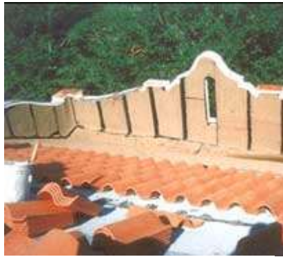
Replacement of damaged clay tile roof.
