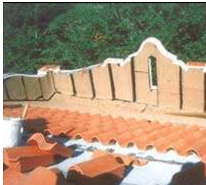
Replacement of damaged clay tile roof.
