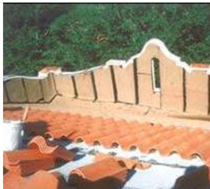
Replacement of damaged clay tile roof.
