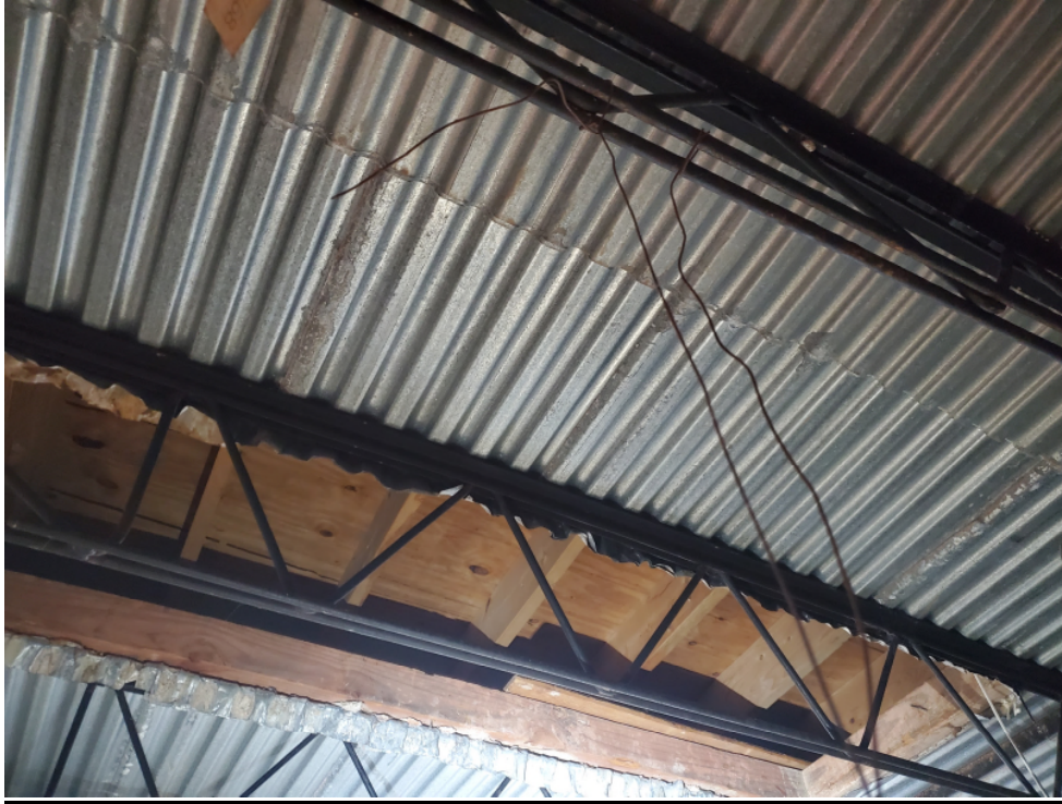
ABOVE CEILING GRID – OPENING IN DECK
