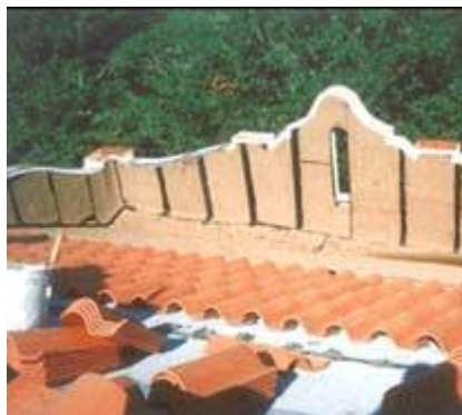
Replacement of damaged clay tile roof.
