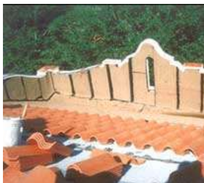
Replacement of damaged clay tile roof.
