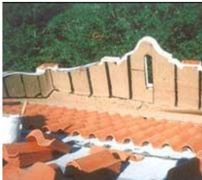
Replacement of damaged clay tile roof.
