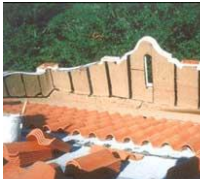
Replacement of damaged clay tile roof.
