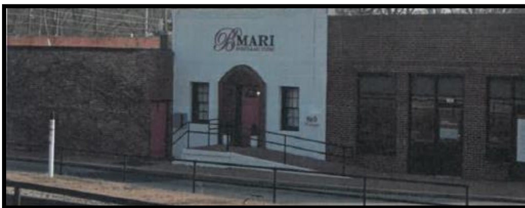
10 - Downtown Block – 106 to 112 North McDonough St.
