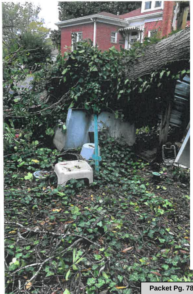
Attachment: Storm Damage (1854 : 145 College Street)
