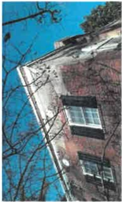
[3] Not Recommended: The white film on the upper corner of this historic brick row house is the result of using a scrub or slurry coating, rather than traditional repointing by hand, which is the recommended method.
